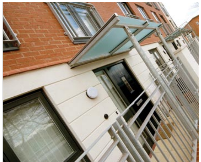
Residential Newbuild Project: Thin Coat EWI System with Ashlar Effect Finish to Ground Floor
