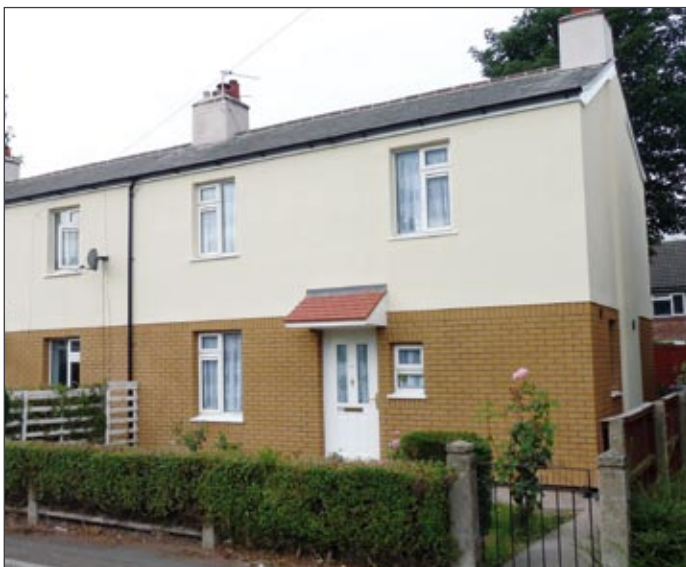
Social Housing Refurbishment Project: Thin Coat EWI System with Brick Effect Finish to Ground Floor & Acrylic Finish to First Floor
